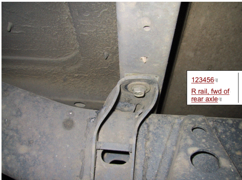
Figure 7. Seat anchorage structure in unitary construction vehicles will typically include both welded and bolted connections. Photograph shows unrepaired accident damage to primary connections which probably makes retrofitting uneconomic.
